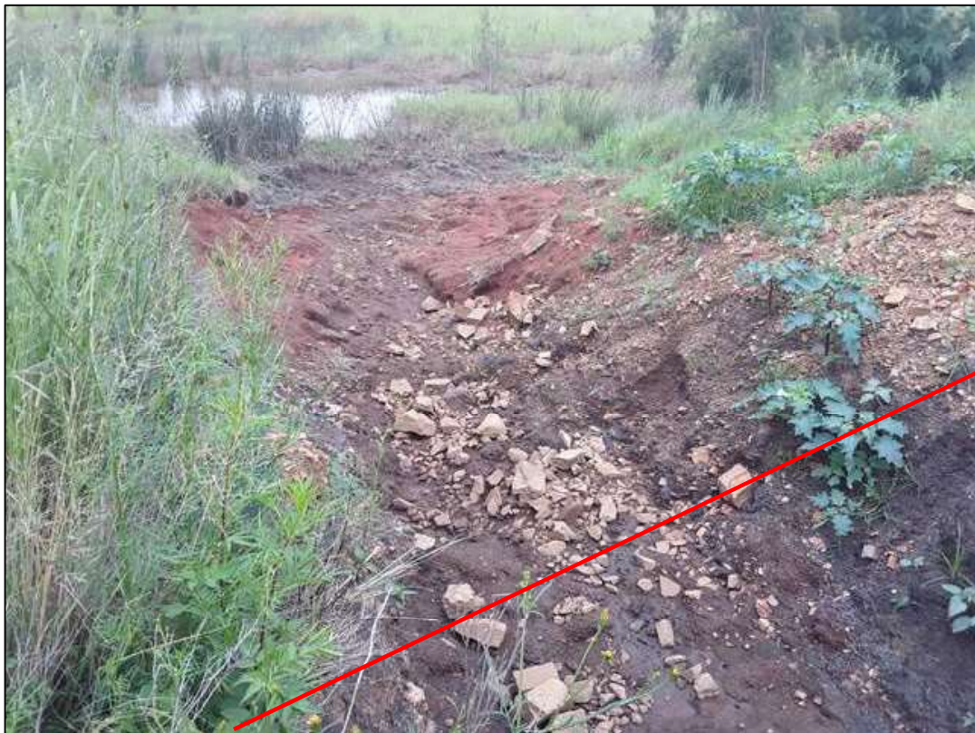
Figure 12: Image of manmade breached section at dividing berm which was necessitates because of high water levels in the LLAWRD (proposed weir position indicated with red line)
