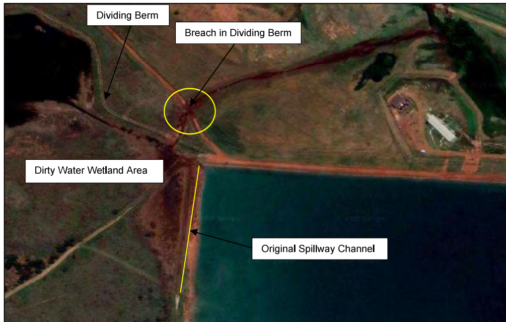
Figure 10: Google Image showing dam's spillway section and dividing berm
