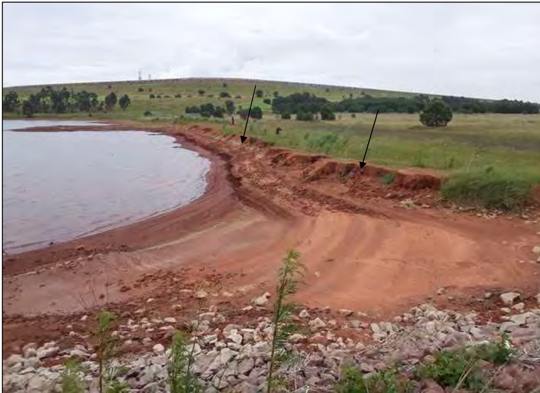
Figure 11: Image of earth berm placed within the original spillway channel
