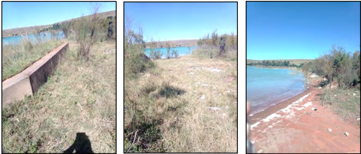
Figure 22. Detail of existing Spillway construction site looking west, southwest and south. Existing structure and retaining wall. (Photos S.M. Miller.)
