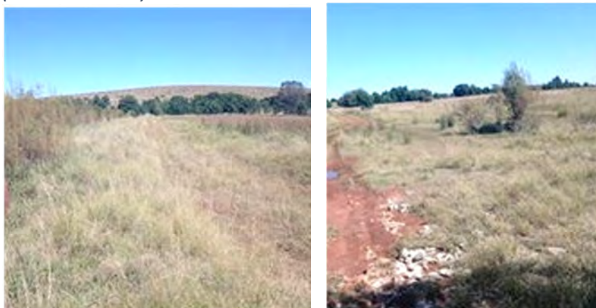
Figure 23. Detail of weir construction site (trench) looking northwest. (Photos S.M. Miller.)
